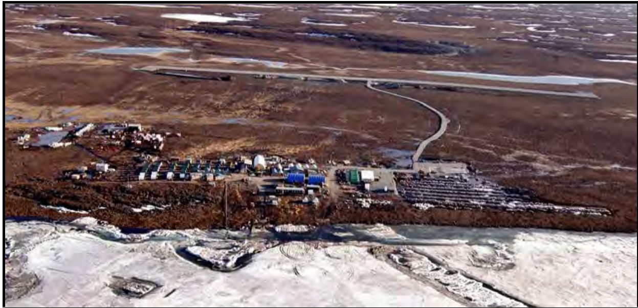
Figure 5.1: Existing Goose Camp (Looking West)
