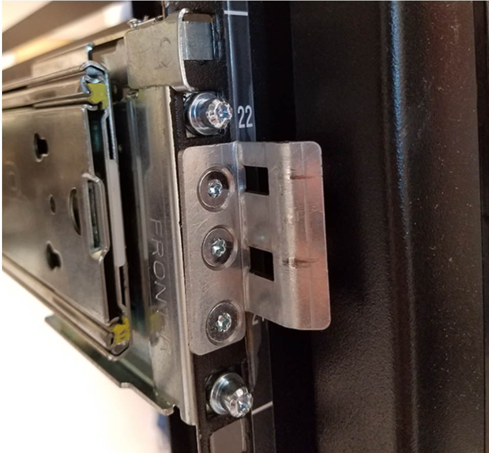
Figure 20: Rack Latch Bracket Installed
