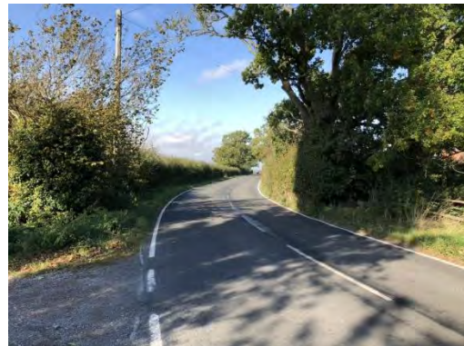
Photograph 4: Conditions on Henfield Road (Westbound)
