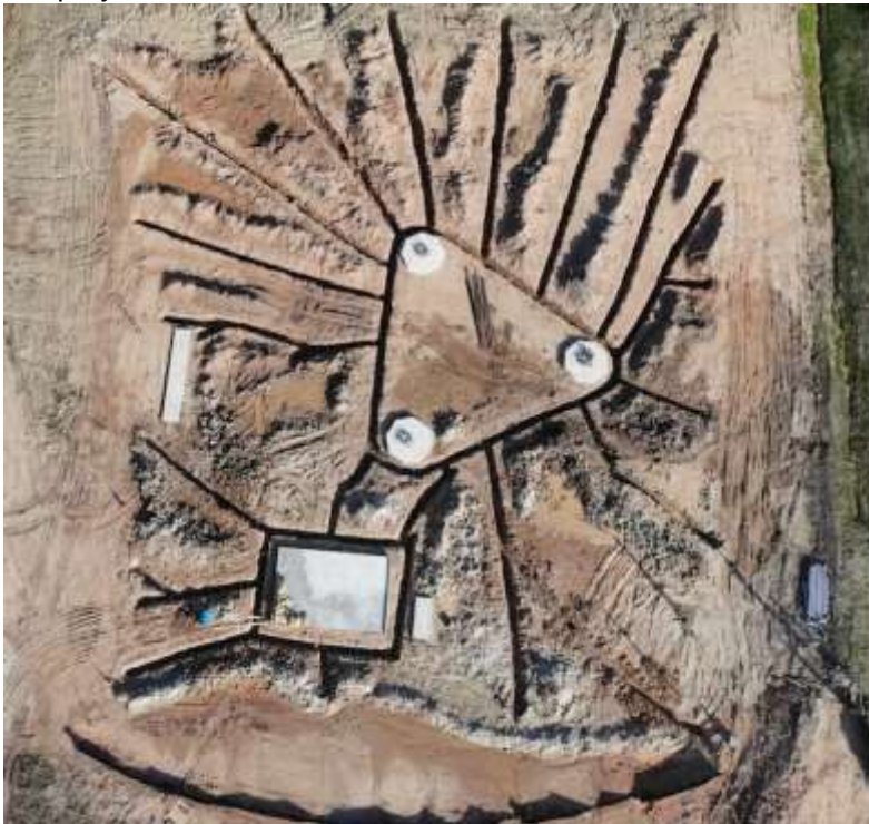
Tower base and grounding phase
