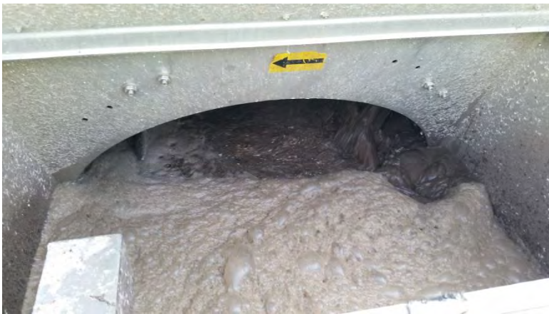
Figure 5 – Flo-beast receiving grease and solids from meat market load
