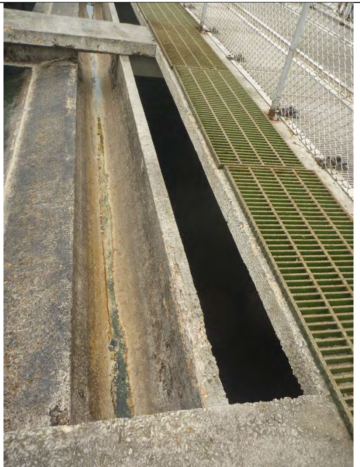
Photo 20 Primary Tank 2 edge of scum trough.
