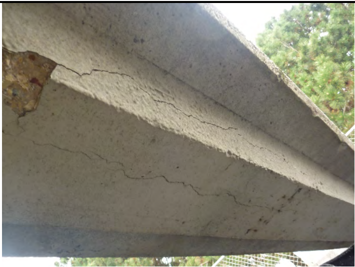
Photo 7 Primary Tank 1 bottom of walkway.
