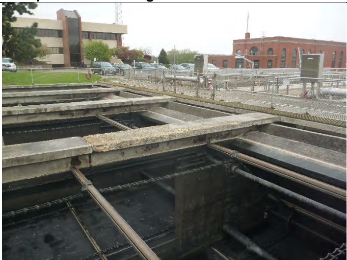
Photo17 Primary Tank 2 bottom of elevated slab, inlet port wall and edge beam.
