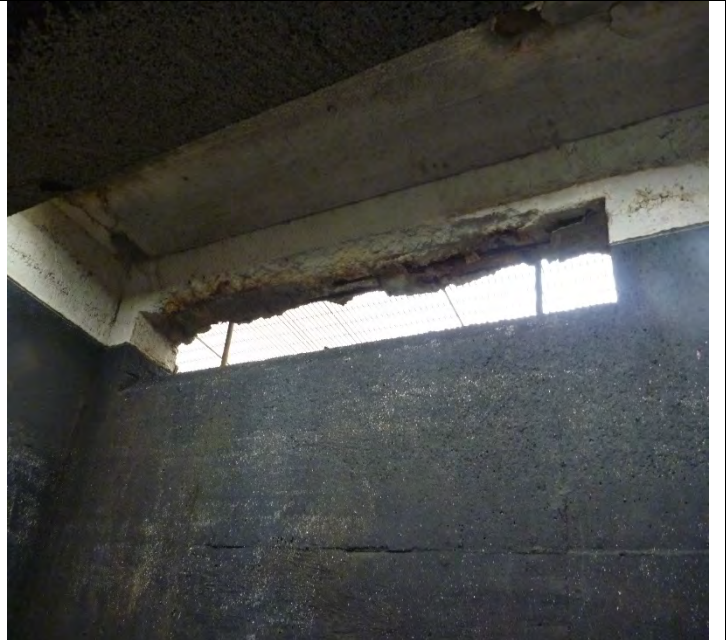
Photo 16 Primary Tank 2 Outlet port wall and slab.
