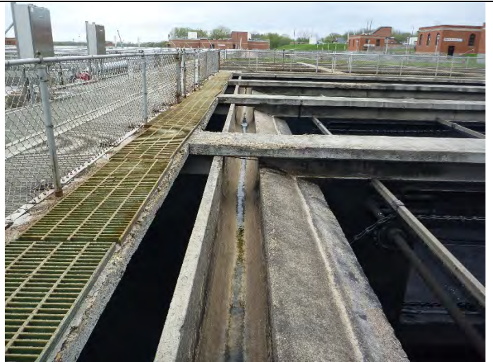
Photo 10 Primary Tank 1 edge of elevated slab.
