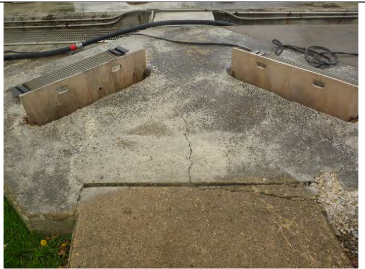
Photo 24 Inlet Structure top surface.
