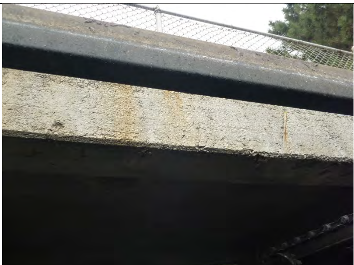
Photo 11 Primary Tank 1 face of edge beam.
