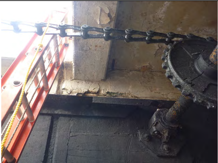
Photo 3 Primary Tank 1 vertical tank walls.
