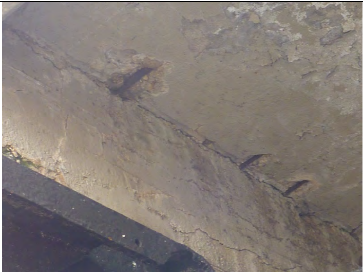
Photo 5 Primary Tank 1 bottom of elevated slab.
