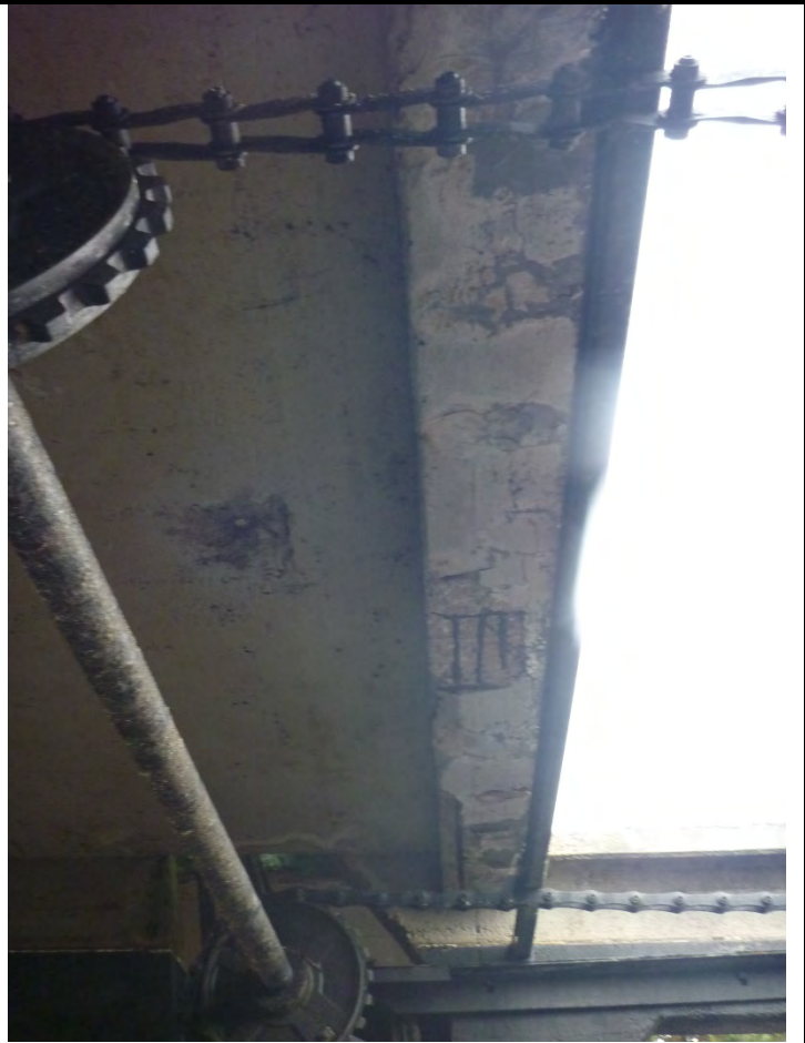
Photo 14 Primary Tank 2 edge beam.
