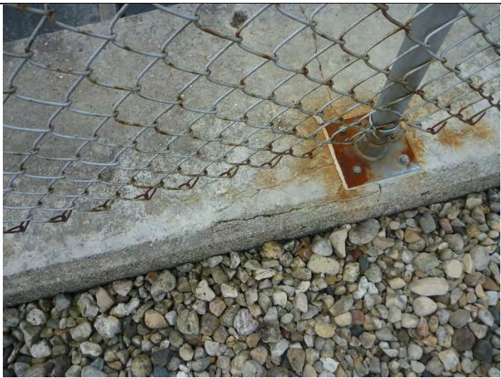
Photo 21 Chain link fence.
