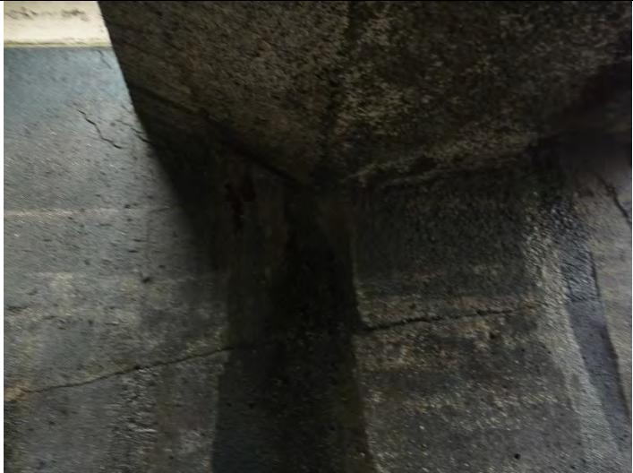
Photo 13 Primary Tank 2 vertical wall crack and delamination at scum trough bearing end.
