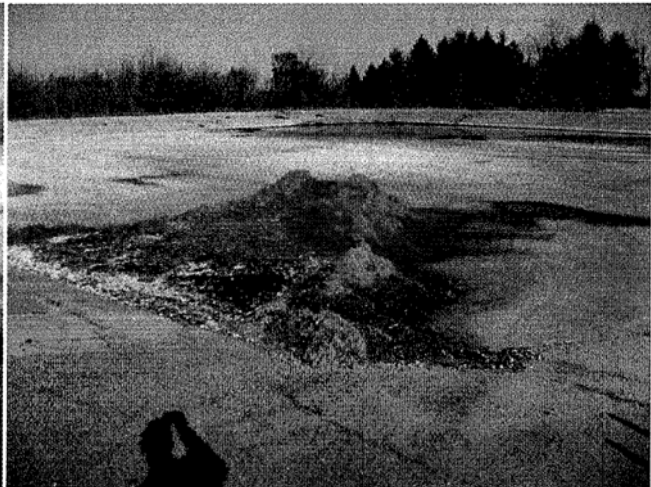
A 79 ton pile of material that had been dumped at the Drying Bed during the Settling Basin waste to Drying Bed trial.
