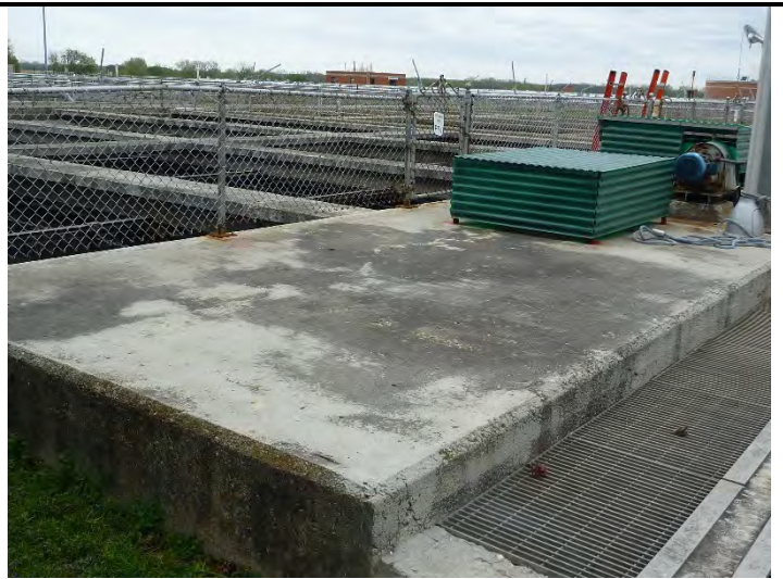
Photo 8 Primary Tank 1 top of elevated slab.
