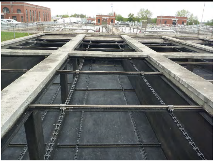
Photo 1 Primary Tank 1 facing north.
