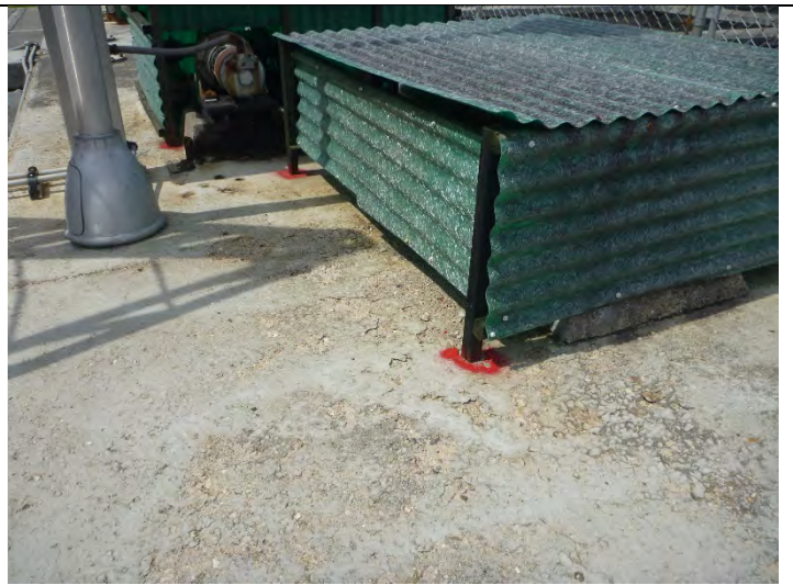
Photo 18 Primary Tank 2 top of elevated slab.
