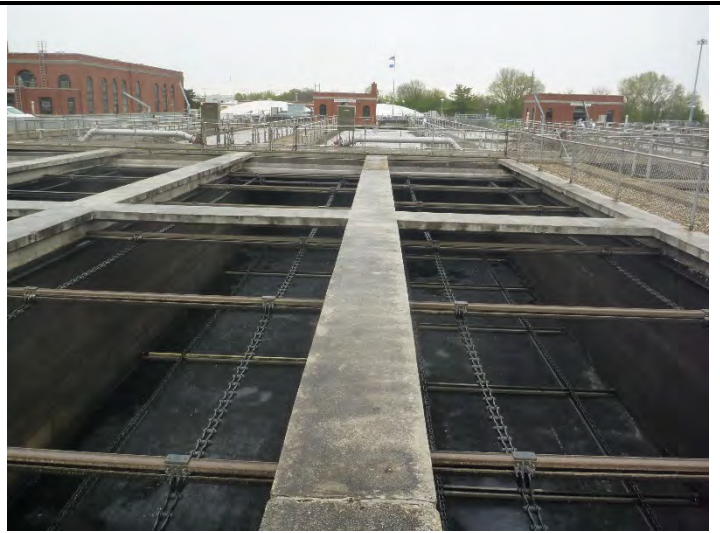
Photo 2 Primary Tank No. 2 facing north.
