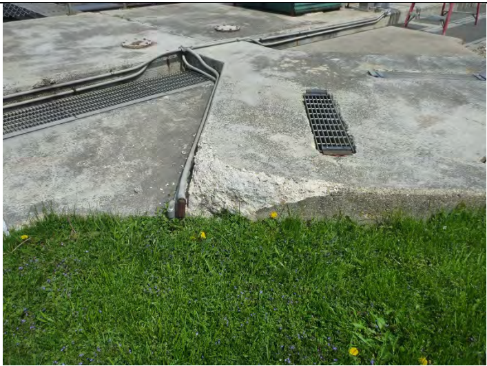
Photo 23 Inlet Structure edge.
