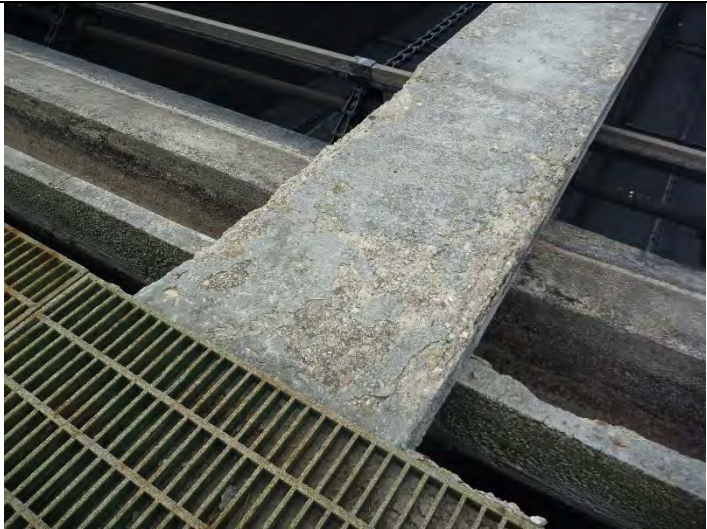
Photo 9 Primary Tank 1 top of walkway.
