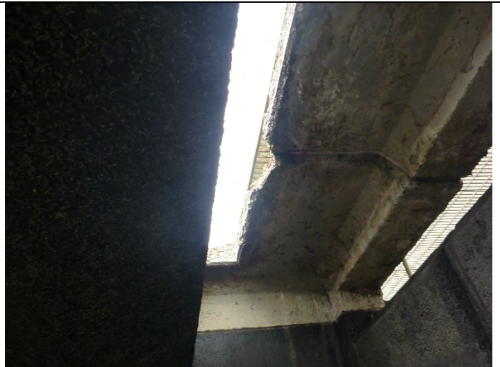
Photo 6 Primary Tank 1 bottom of elevated slab.
