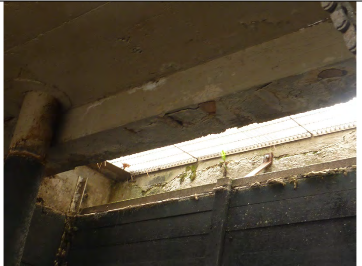
Photo 4 Primary Tank 1 elevated slab edge beam.
