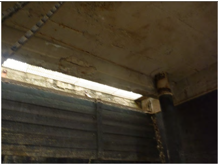
Photo17 Primary Tank 2 bottom of elevated slab, inlet port wall and edge beam.
