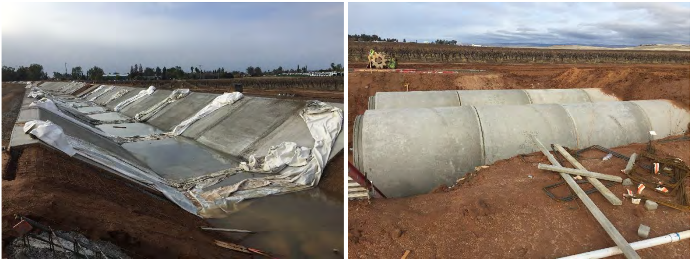
Tesoro Viejo Project: Lat. 6.2 Concrete Canal Lining and dual 84” Pipeline Construction
