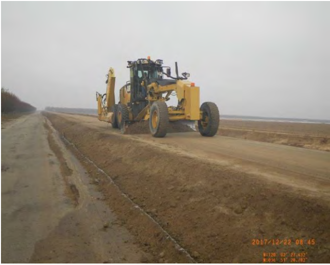
16.9 Graded and Sloped West of Rd. 28
