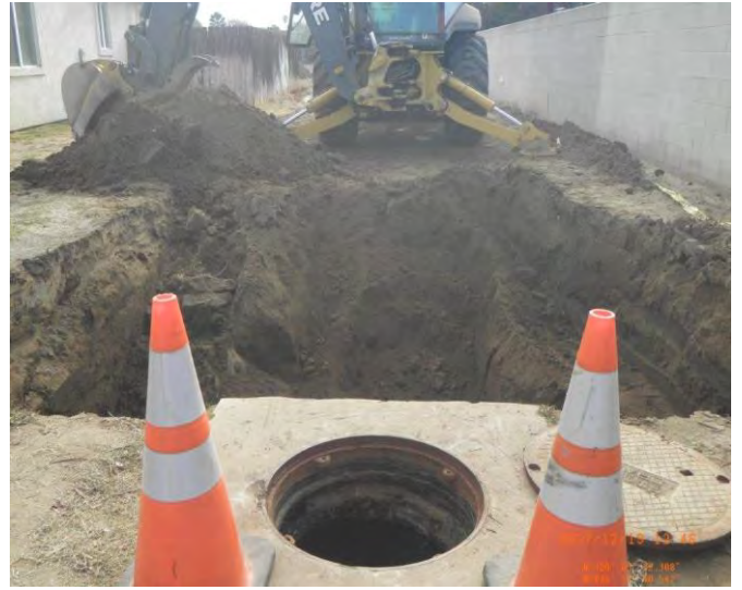
Roberts Alleyway Pipeline Leak Repair
