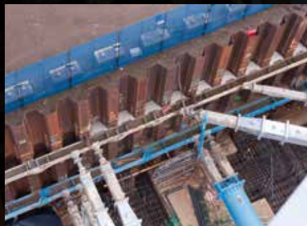
Trench Sheets & Sheet Piles
