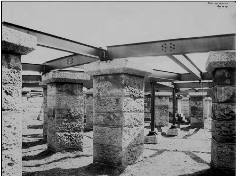
Two photos captured in 1897 show the steel foundation for the basement floor in place at the state Capitol. Hidden behind walls for decades, this foundation area is now the L'Etoile du Nord Vault, Room B15, which is a new space for public meetings and gatherings.
