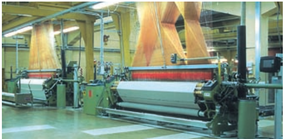
DORNIER-rapier weaving machine installation at the Zucchi plant in Casorezzo
