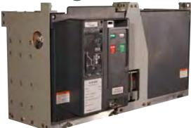
The Leonardo DRS 4040 is a 2400-4000A low voltage Air Circuit Breaker utilizing the latest technology electronic trip unit. This circuit breaker is based on a COTS breaker that is militarized by DRS providing a small, lightweight, and cost effective solution. Utilized on the latest U.S. Navy ships for power distribution, the military hardened air circuit breaker is designed to withstand rugged maritime conditions for the life of the ship.
