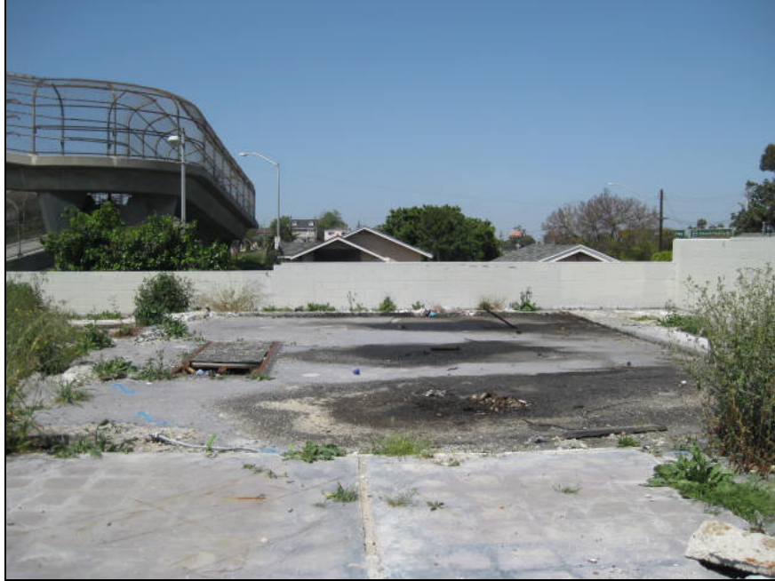
Photo 5: Photo facing north. Note the staining on the concrete pad where the hoists are located. The clarifier is located in the northeast corner of the concrete pad.
