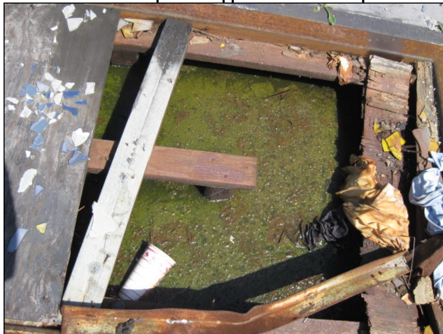
Photo 8: Close-up of the apparent oil/water separator.
