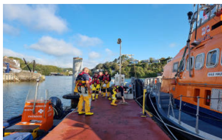
Work on the pontoons
