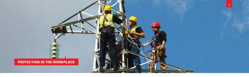
For work in a single place of work with protection by means of a rope with brake, a fall absorber or a retractable system. For simultaneous positioning by means of a positioning device.
