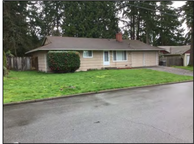
Figure 7-26. 13028 109 th Ave. NE, view southeast.
