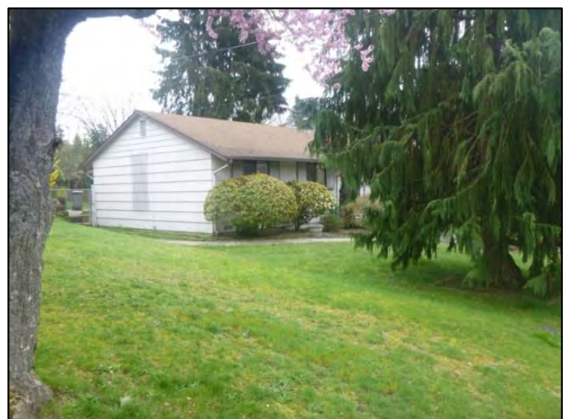
Figure 7-46. 12814 109 th Ave. NE, view southeast.
