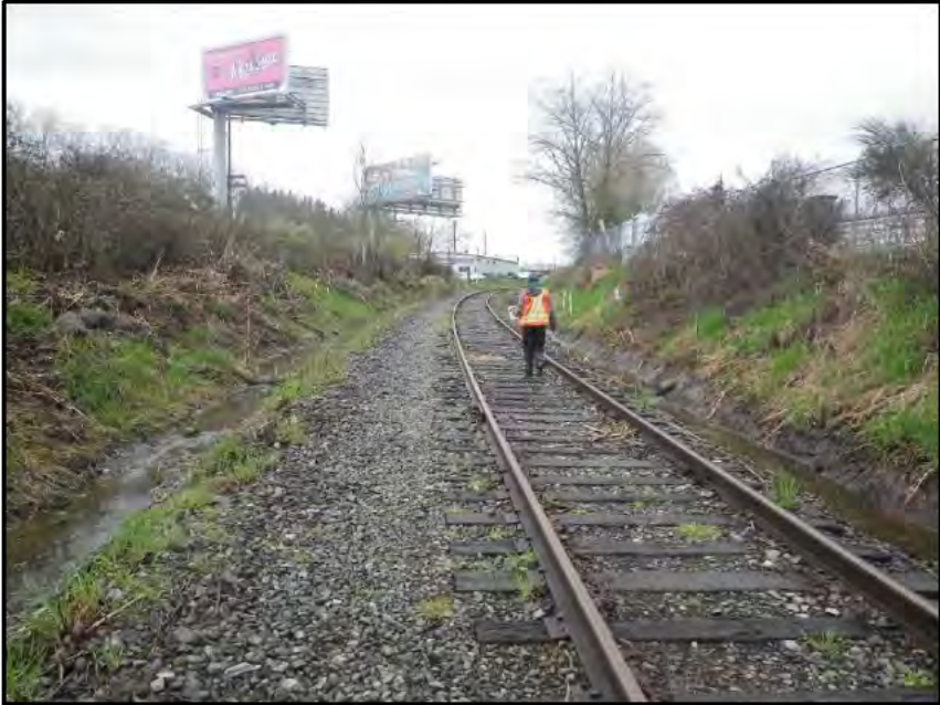
Figure 7-4. Survey along the abandoned, intact railroad line on rerouted segment of the alignment north of pole 2/4, view west.
