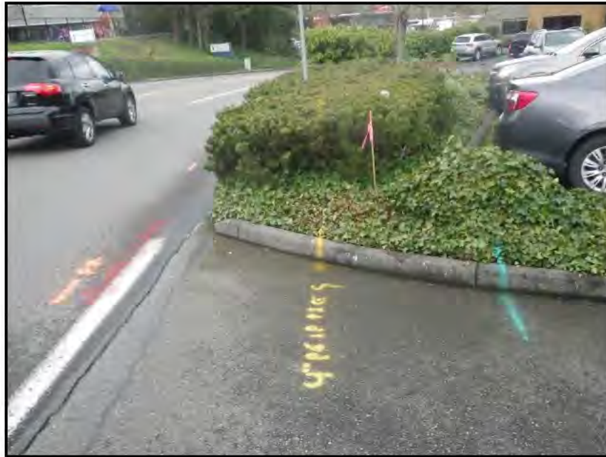
Figure 7-2. Staked location of Pole 3/15, along 120 th Ave. NE, view west. Note utility locate markings indicating an existing gas line ( yellow ) and sewer line ( green ) adjacent on either side of the proposed pole location. Buried communication ( orange ) and power ( red ) lines are also indicated at the edge of the roadway, south of the proposed pole location.
