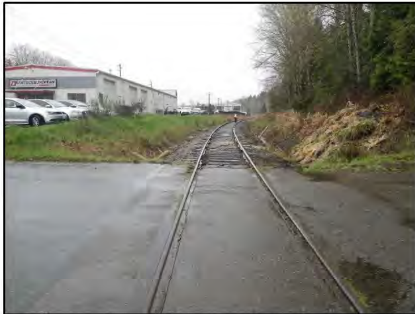
Figure 7-15. Segment of Site 45KI1274 with intact rails and ties, view west. Note asphalt street crossing in foreground.
