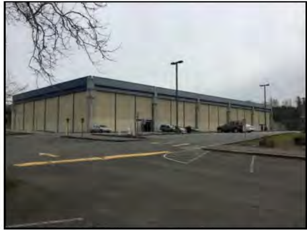
Figure 7-23. The gymnasium at 10601 NE 132 nd St., view southeast.
