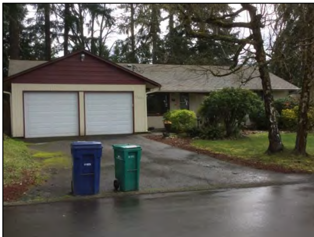
Figure 7-27. 13020 109 th Ave. NE, view southeast.
