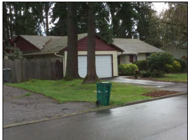
Figure 7-28. 13020 109 th Ave. NE, view southeast.
