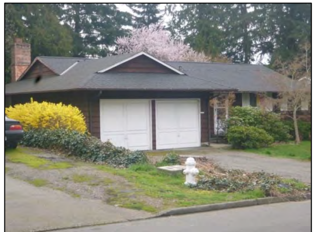
Figure 7-40. 12836 109 th Ave. NE, view southeast.
