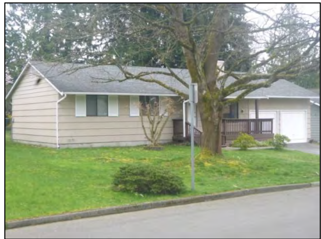
Figure 7-42. 12830 109 th Ave. NE, view southeast.
