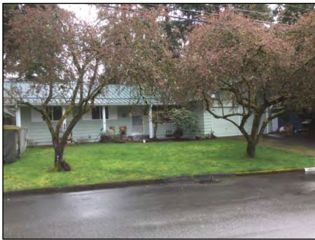
Figure 7-29. 13012 109 th Ave. NE, view southeast.
