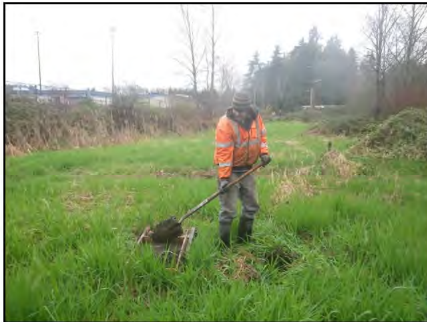
Figure 7-7. Adam Fruge excavating SP 6 ( Pole 4/10 ), view northwest.
