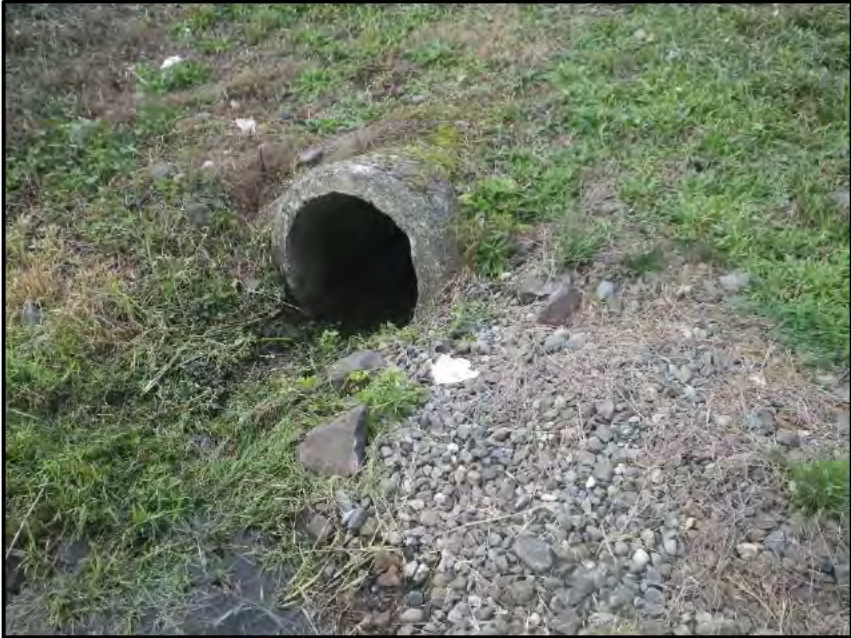
Figure 7-14. Cylindrical concrete pipe culvert at base of railroad berm in new segment of Site 45KI451, view southwest.
