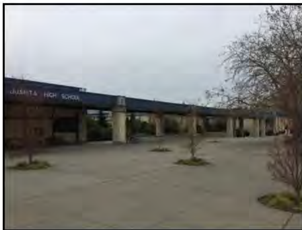
Figure 7-20. 10601 NE 132 nd St., view southwest
