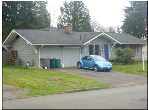
Figure 7-44. 12822 109 th Ave. NE, view southeast.
