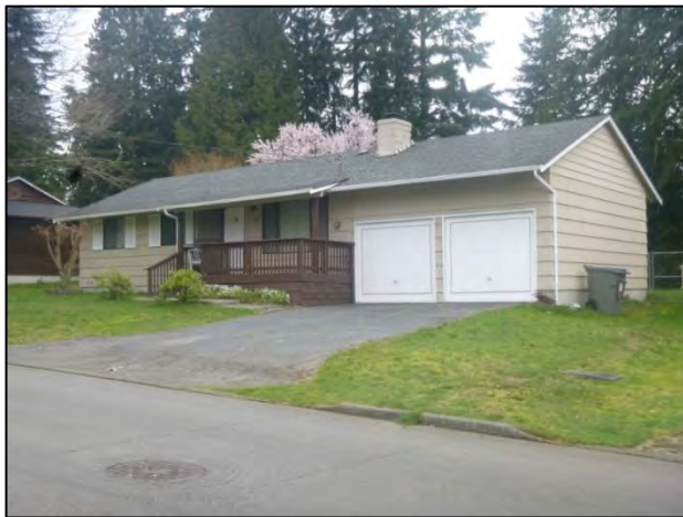
Figure 7-41. 12830 109 th Ave. NE, view northeast.
