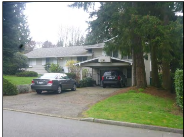
Figure 7-36. 12852 109 th Ave. NE, view northeast.
