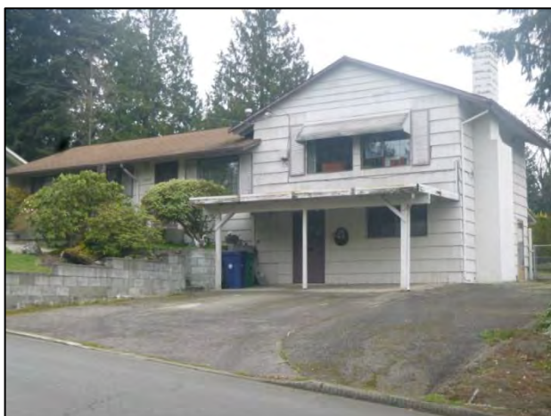
Figure 7-45. 12814 109 th Ave. NE, view northeast.
