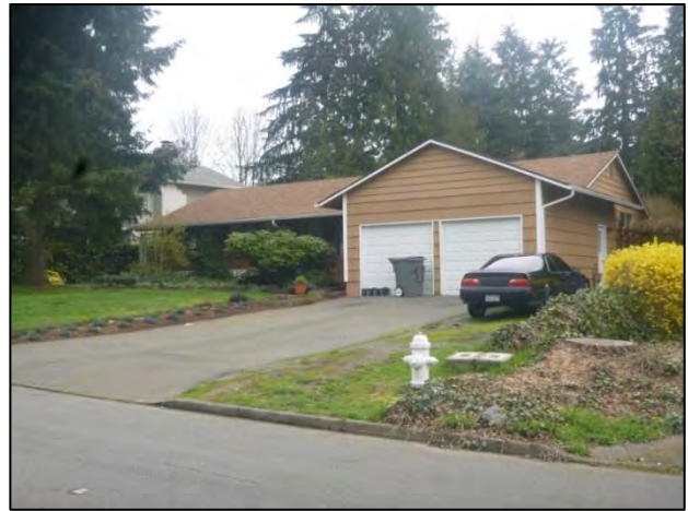
Figure 7-38. 12844 109 th Ave. NE, view northeast.
