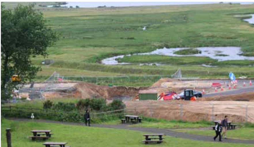
The underpass under construction
