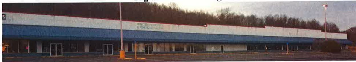
Right Side of Building
