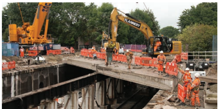
The bridge deck was made up of approximately 80 steel and concrete beams, each 18 metres long
