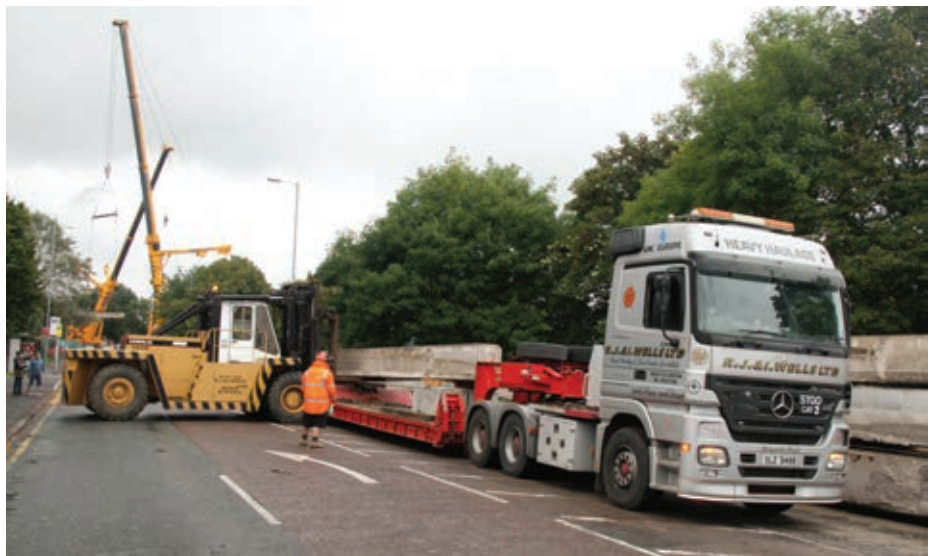
The bridge deck was made up of approximately 80 steel and concrete beams, each 18 metres long
