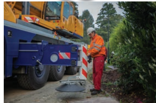
Additional steel plates were placed at the site ready for the crane's outriggers
