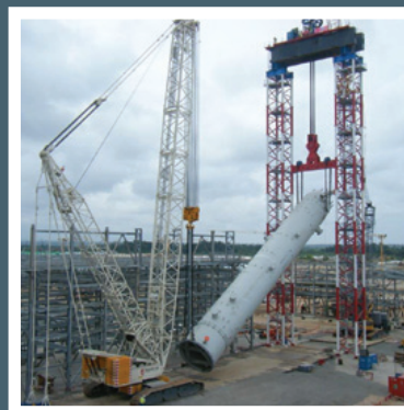
TEREX DEMAG CC2800-1, 600 ton capacity
