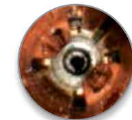
A Hawkeye Pro MicroFlex Semi-Rigid borescope inspecting a very small electrical socket
