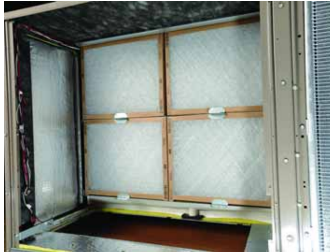
Figure 15: Bottom Return Opening For Side Duct Conversion
