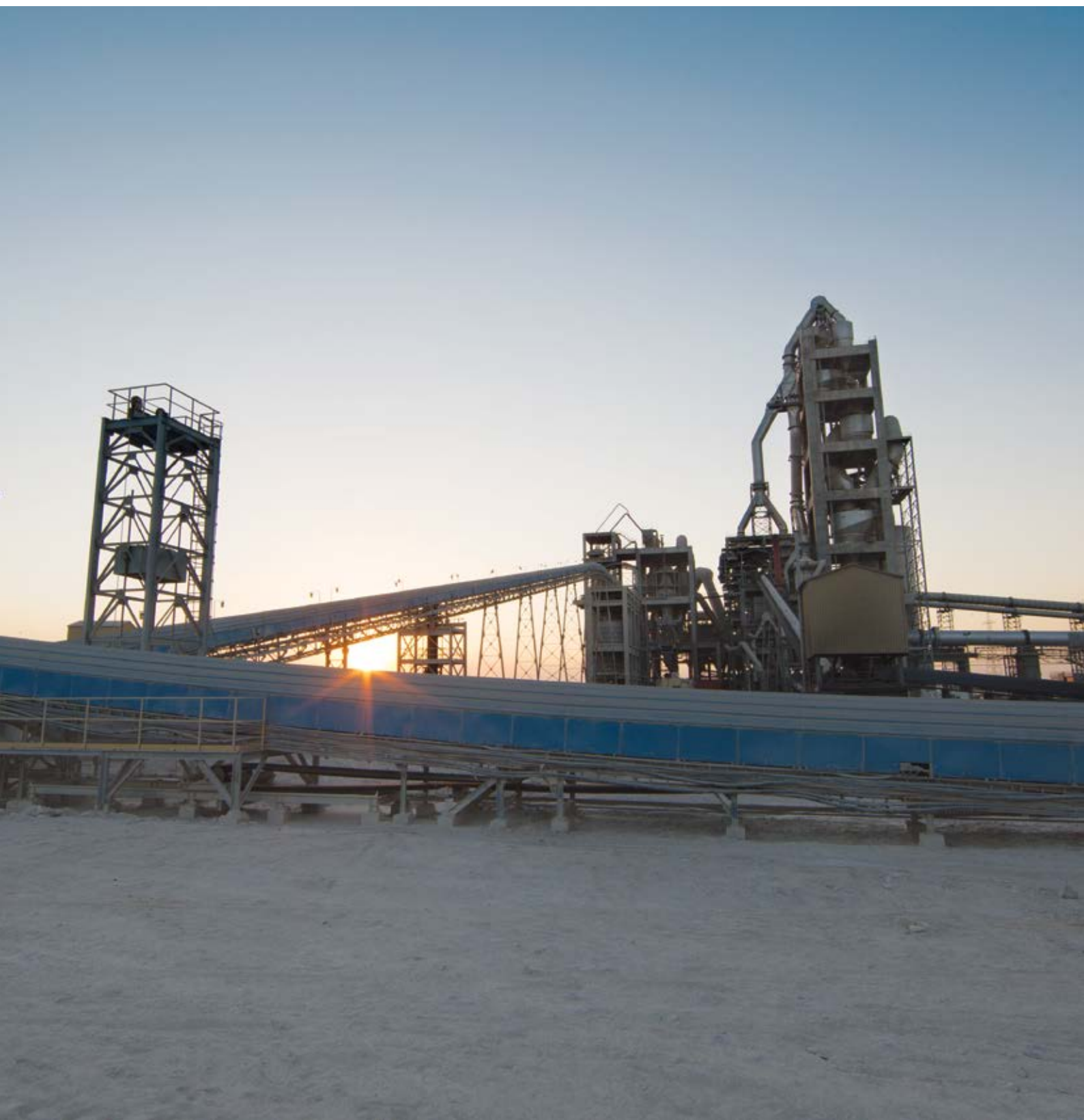
➤ View of the preheater, Mangrol
