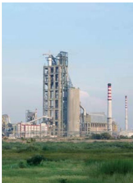
➤ A View of Muddapur Plant, Karnataka
