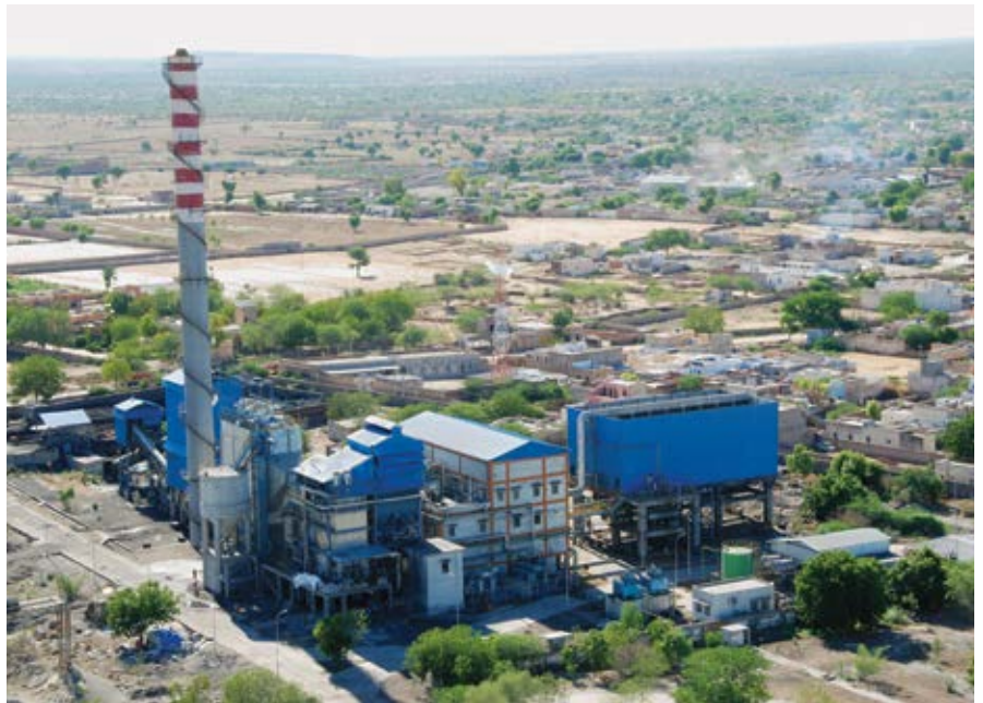
▶ A View of Power Plant at Gotan, Rajasthan
