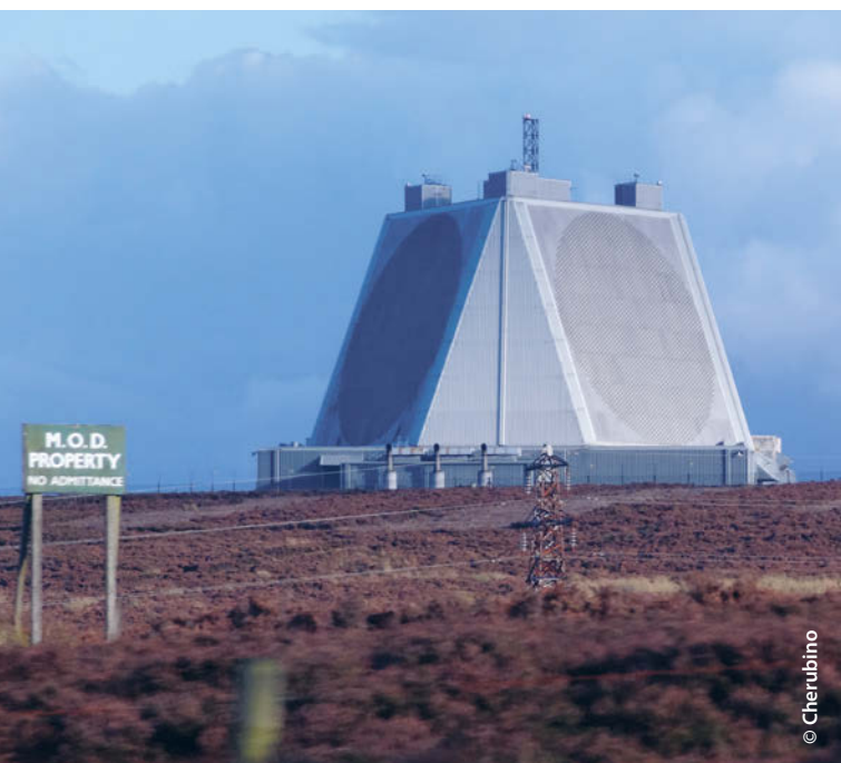
Solid State Phased Array Radar (SSPAR) at RAF Fylingdales, North Yorkshire, UK.
