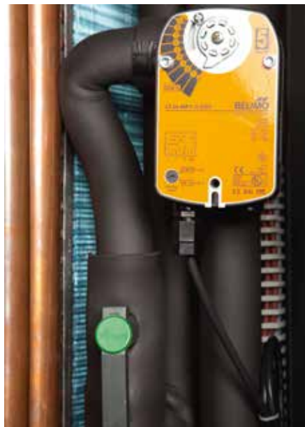
Switchover between a 2 and 3-way valve
