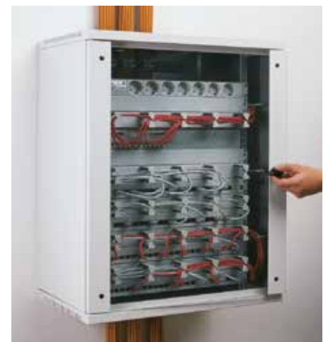
6. Installation is now complete.
