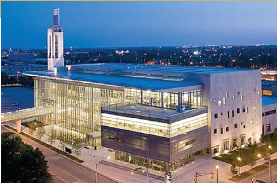
Campus Center, IUPUI
