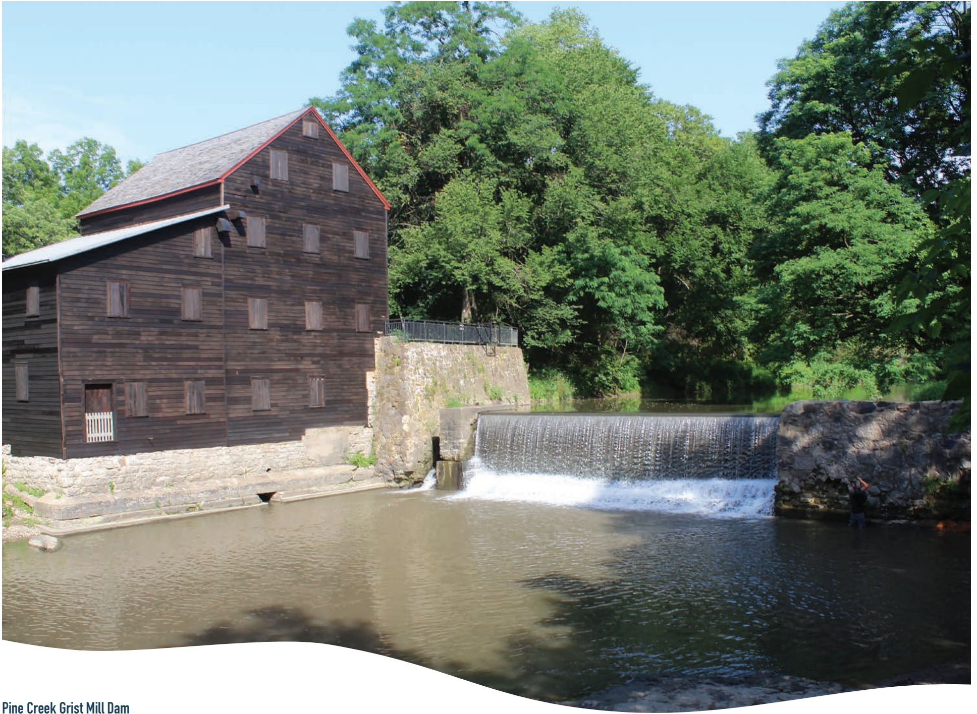
Pine Creek Grist Mill Dam
