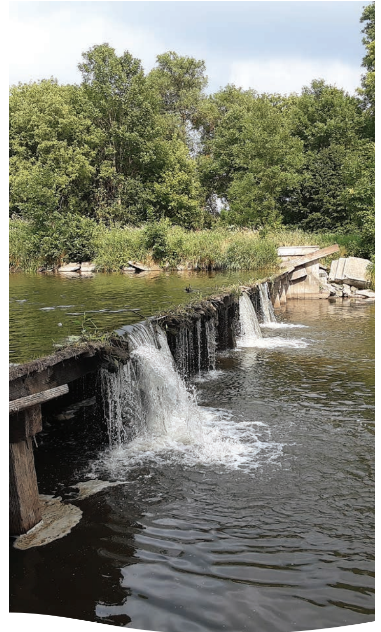
Ashton Dam Osceola County
