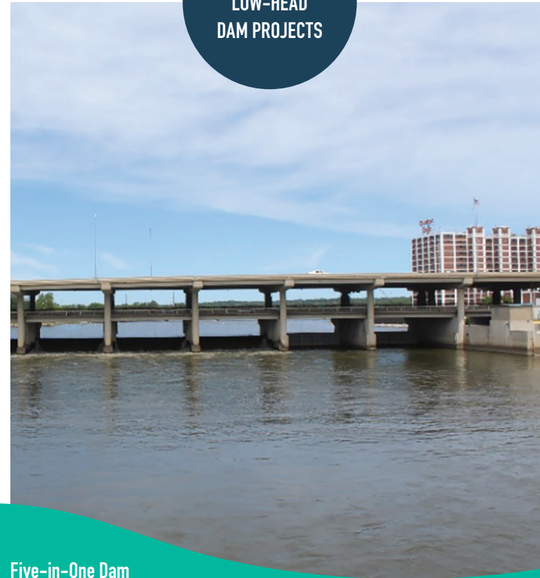
Five-in-One Dam Linn County
