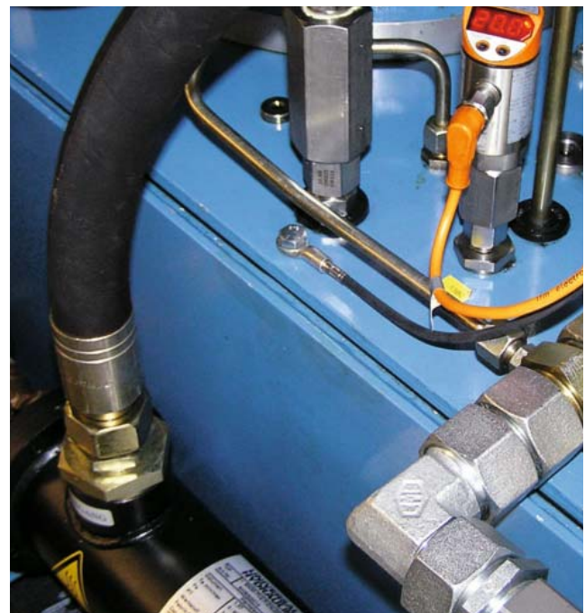
Pt100 temperature sensor attached to an oil tank to monitor the housing temperature.
