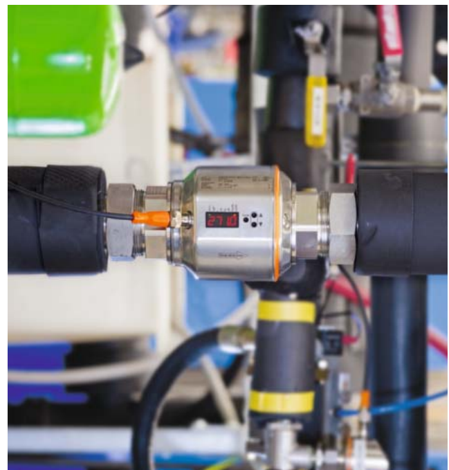
Magnetic-inductive volumetric flow sensor for measuring the water quantity in a filtration system.
