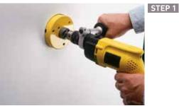
Determine location and cut hole in wall using hole saw, keyhole saw or a core drill.
