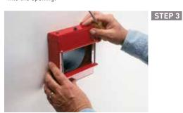
Place the FlameStopper Thru-Wall fitting box over the opening and secure the two bolts.
