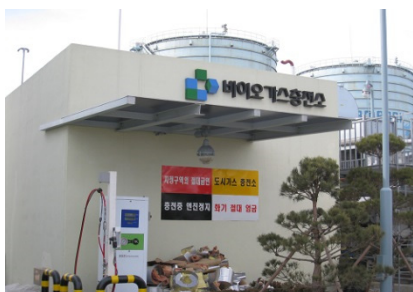
Fig. 1 Biomethane Charging Station
