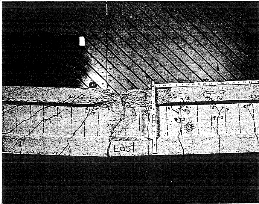
FIG. 55 FLEXURAL FAILURE IN A BEAM WITH EIGHT WIRES
