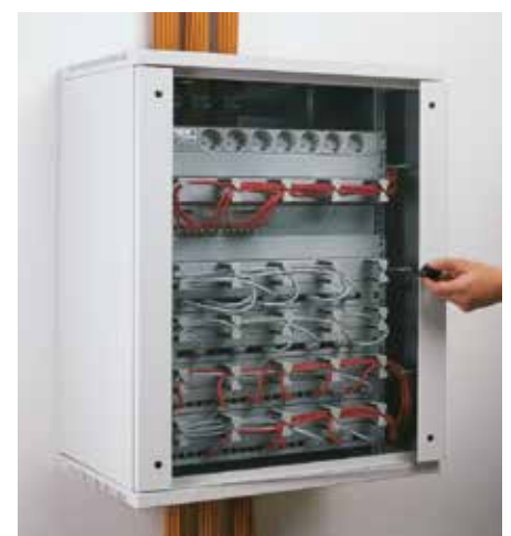
6. Installation is now complete.
