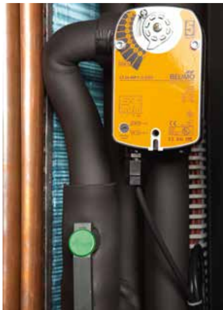
Switchover between a 2 and 3-way valve
