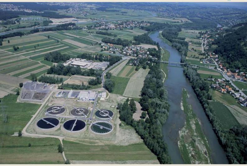
Many of the municipal sector improvements in Danube countries are only now starting to be realised. Tertiary treatment (nitrogen and phosphorus removal) is being applied for a large number of the upgraded and new wastewater treatment plants. Furthermore, demands for nitrogen and phosphorus removal for wastewater treat-
