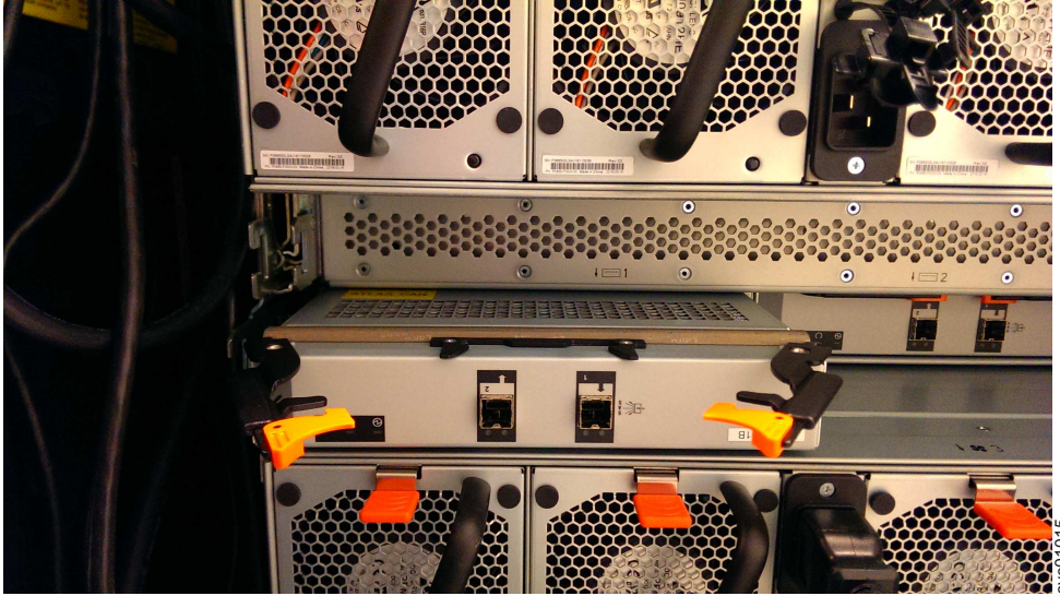
Figure 77. Removing the expansion canister
