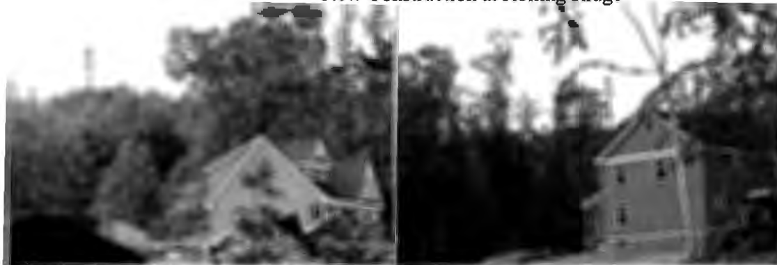
New Construction at Rolling Ridge
