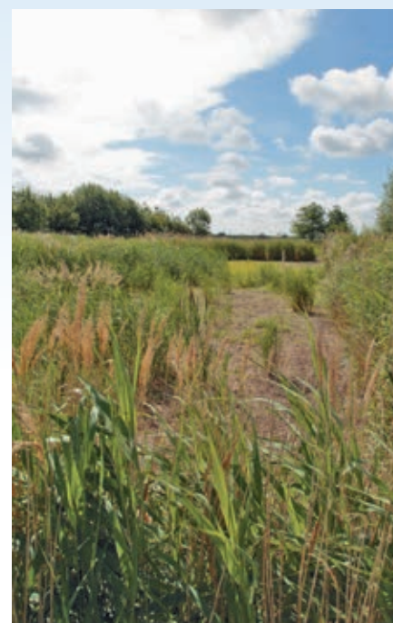
The reed bed water treatment facility at Produce World Yaxley.
