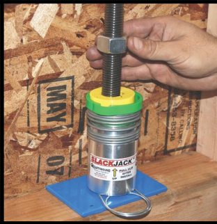
Place color coded washer and spin nut down hand tight.
