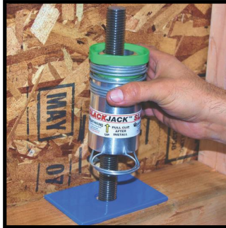
Slide Slackjack® on top of color bearing plate.
