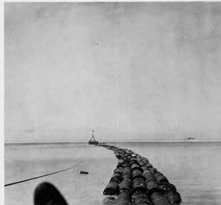
Floating Outfall Line
