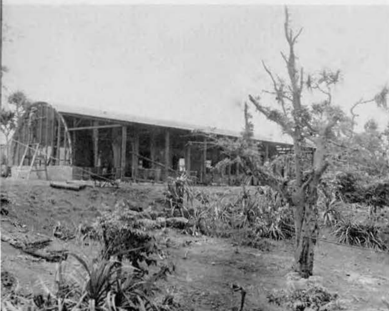
OFFICERS' MESS CONSTRUCTION
