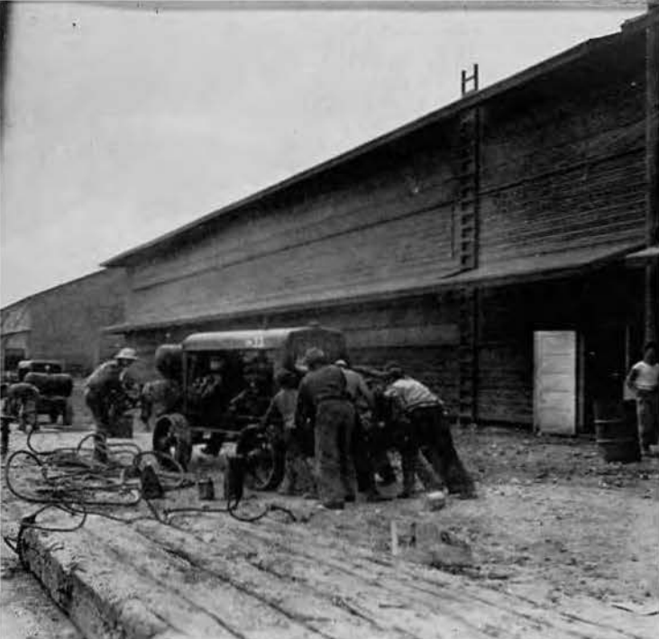
Excavating for Main
