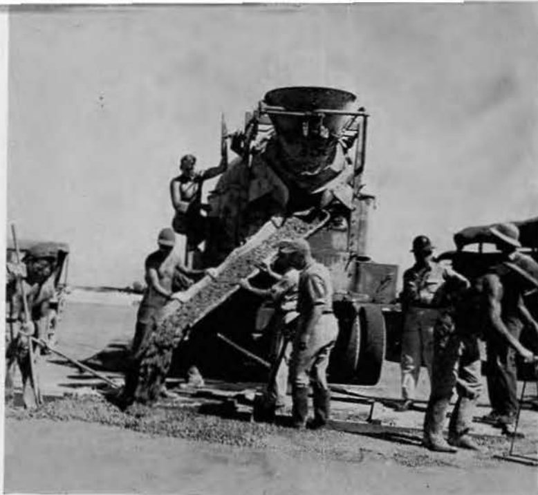
Placing Concrete Slab
