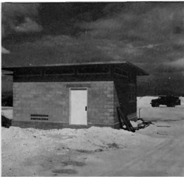
Control Building at Tank Farm
