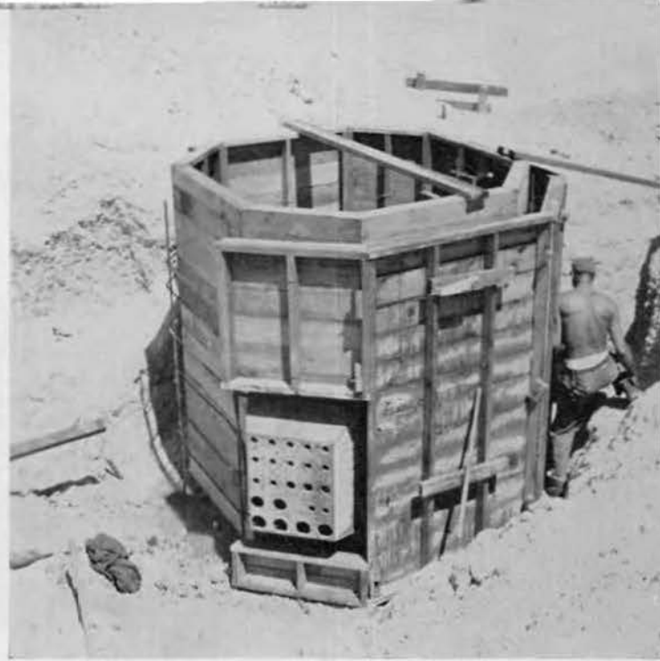
Electric Manhole
