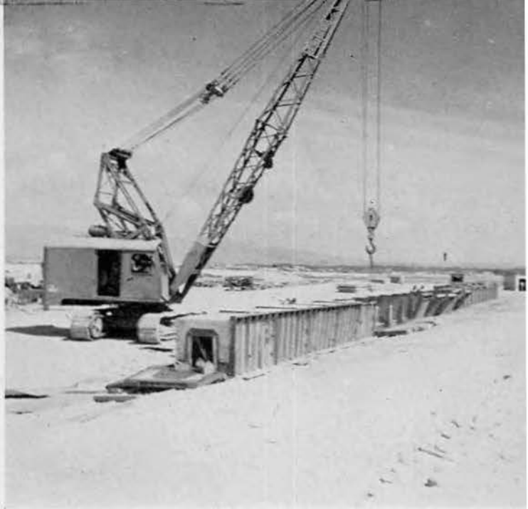
Stripping Precast Culvert Forms
