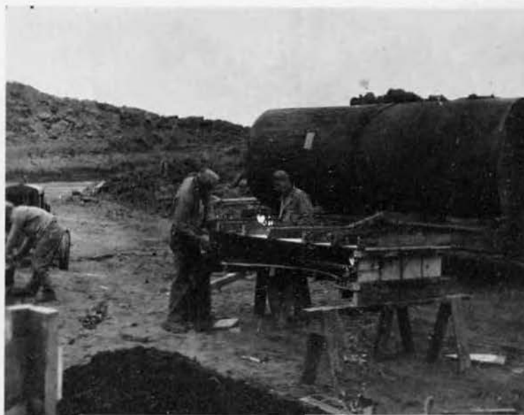
PLACING DIESEL TANKS
