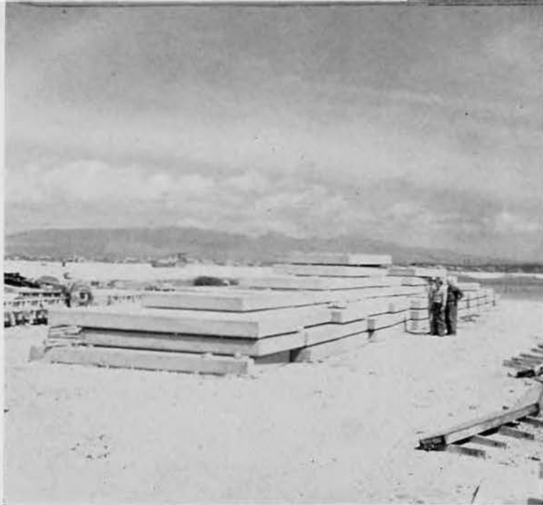
Precast Concrete Slabs for Seaplane Ramp
