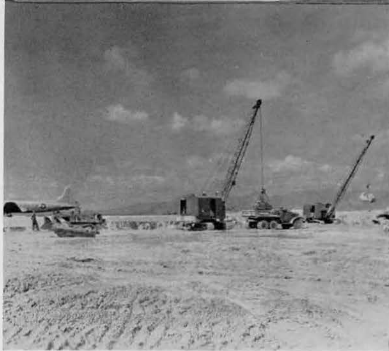
Excavation for Back Fill
