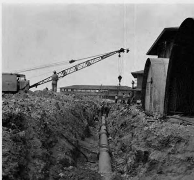
12-inch Main in Place
