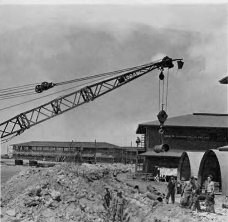
Laying 12-inch Main
