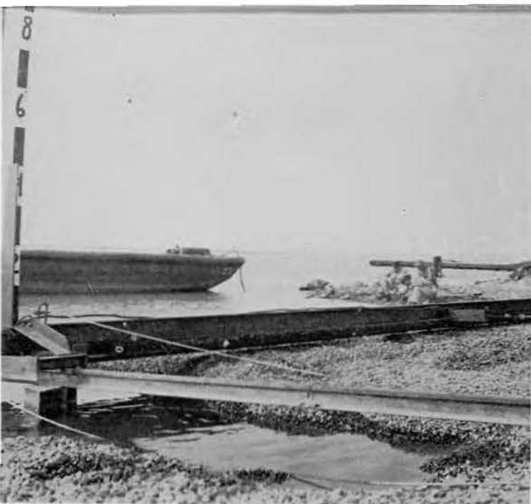
Sub-Grade Screeding Rail in Place
