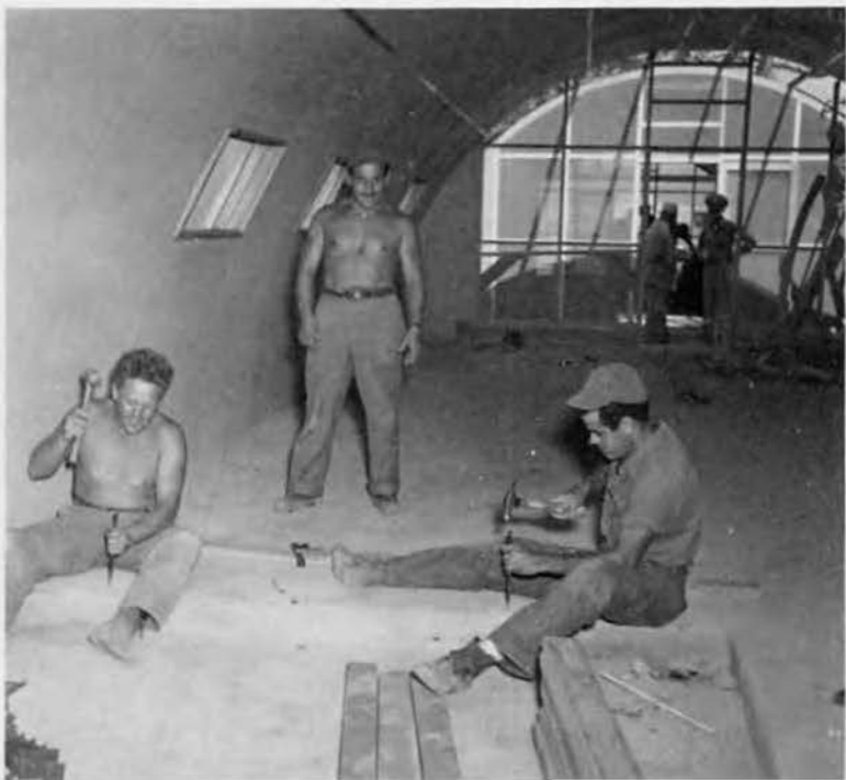
Interior of Quonset
