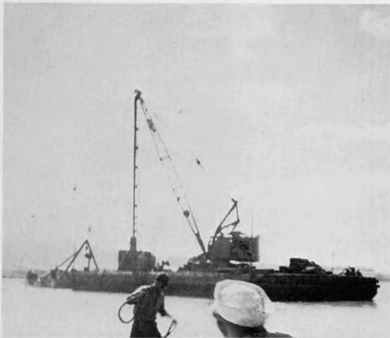
Pile Driving Barge
