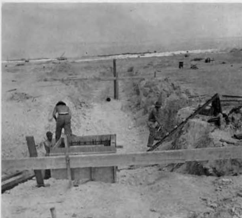
Storm Drain Manhole
