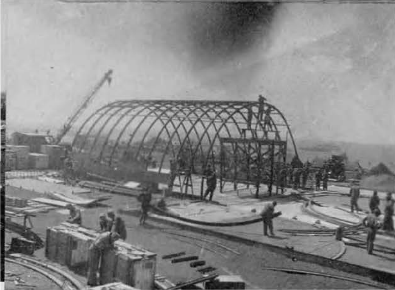
RIBS GOING UP
