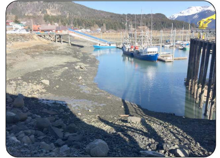
C DREDGE AREA (C) LOOKING NORTH
