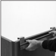
Install accessories with metal support (pencil tray, rail, shelf) at the right height before installing the next stackable panel.
