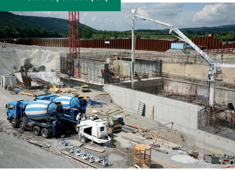
Concrete output max. 95 m³/hr
