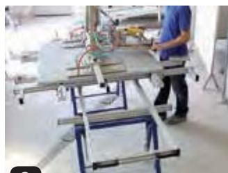
2 loading of slabs
