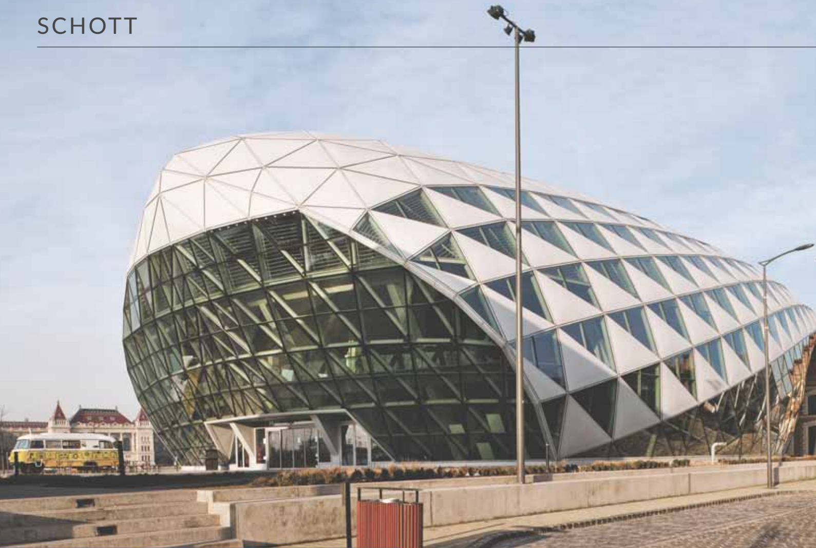
The Bálua Budapest center is known simply as “the whale” to the locals. It is equipped with fire-resistant PYRAN® glass.
