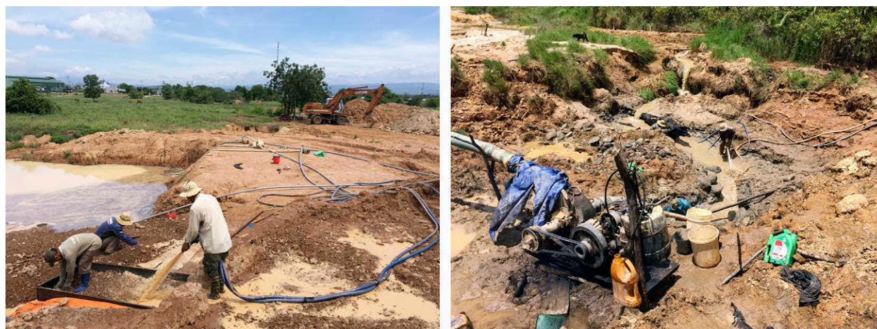
Figure 4. In areas mined with machinery, backhoes were used to remove topsoil and reach the gem-bearing gravel layers prior to washing and sieving using a water pump in the gem fields of Binh Thuan (left) and Krong Nang (right). Photos by Doan Thi Anh Vu.
