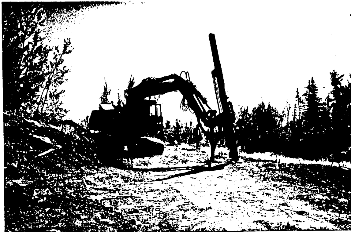
1280-MOUNTED HYDRAULIC DRILL WORKING IN SECTION F
