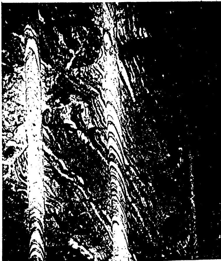
CLOSE-UP OF UNWEATHERED CLEAN FACE EXPOSED BY PERIMETER DRILLING IN SECTION G
