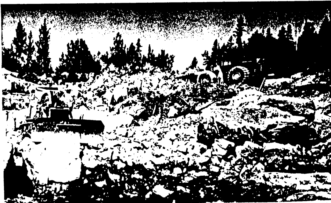
992 CAT LOADER AND D-6 DOZER PUSH STRIPPED OVERBURDEN TO EXTREMITIES OF MAIN DEPOSIT
