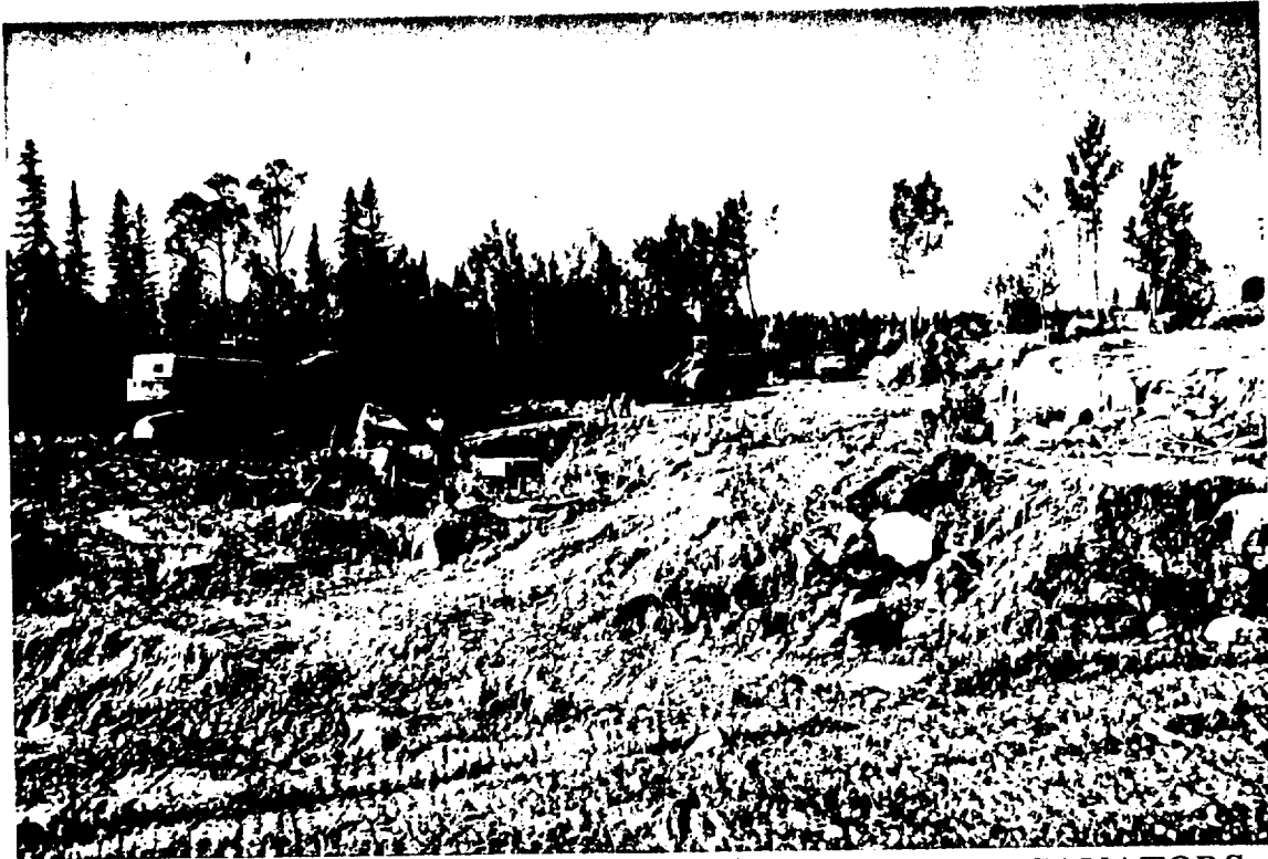
STRIPPING IN PROGRESS, USING 220-B AND 170-C EXCAVATORS, 992 CAT LOADER, SERVICE TRUCKS AND MECHANIC'S TRUCK
