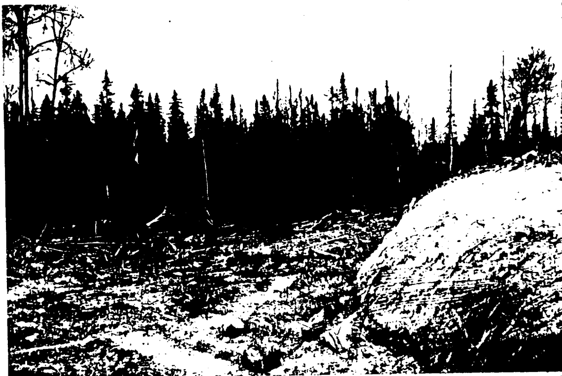
"CLEARING AND GRUBBING" UNDERWAY PRIOR TO EARTH EXCAVATION
