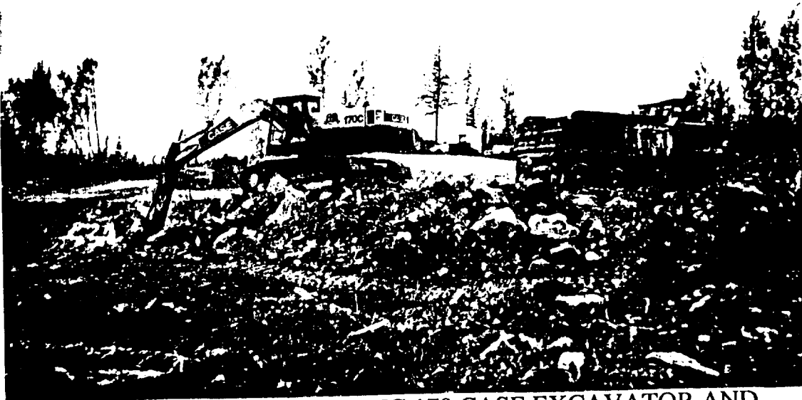
STRIPPING CREW EMPLOYING 170 CASE EXCAVATOR AND RED TRIAXLE MACK DUMP TRUCK
