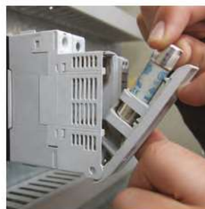
3. Removal or Insertion of fuse
