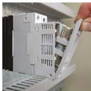
2. Opening or closing the fuse holder
