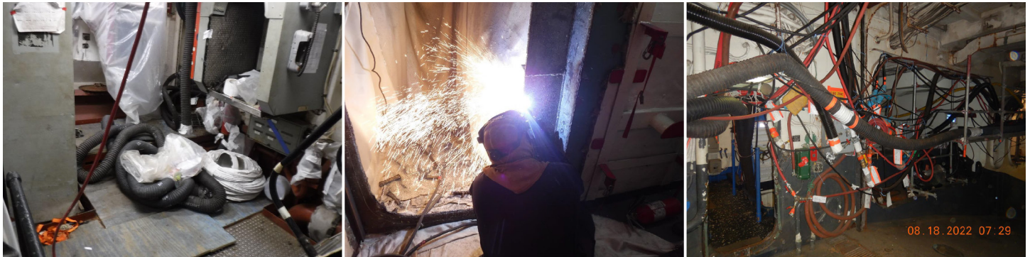
Figure 4: Fire Risks aboard Ships Undergoing Maintenance
