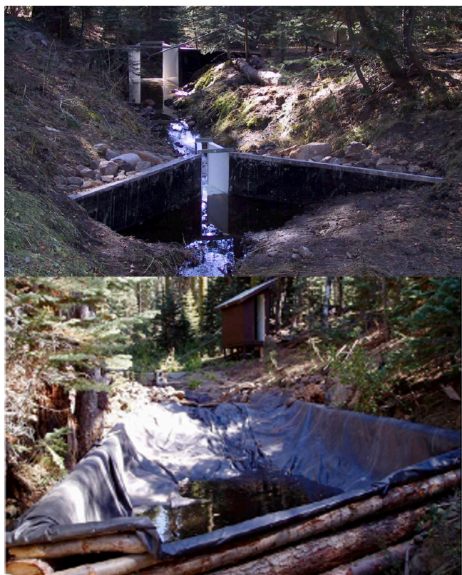
Fig. 3. Parshall Montana flumes, small flume in the foreground and large flume in the background, looking downstream, in B201 (top). An empty sediment pond with pond liner and log structure, looking upstream in B204 (bottom).
