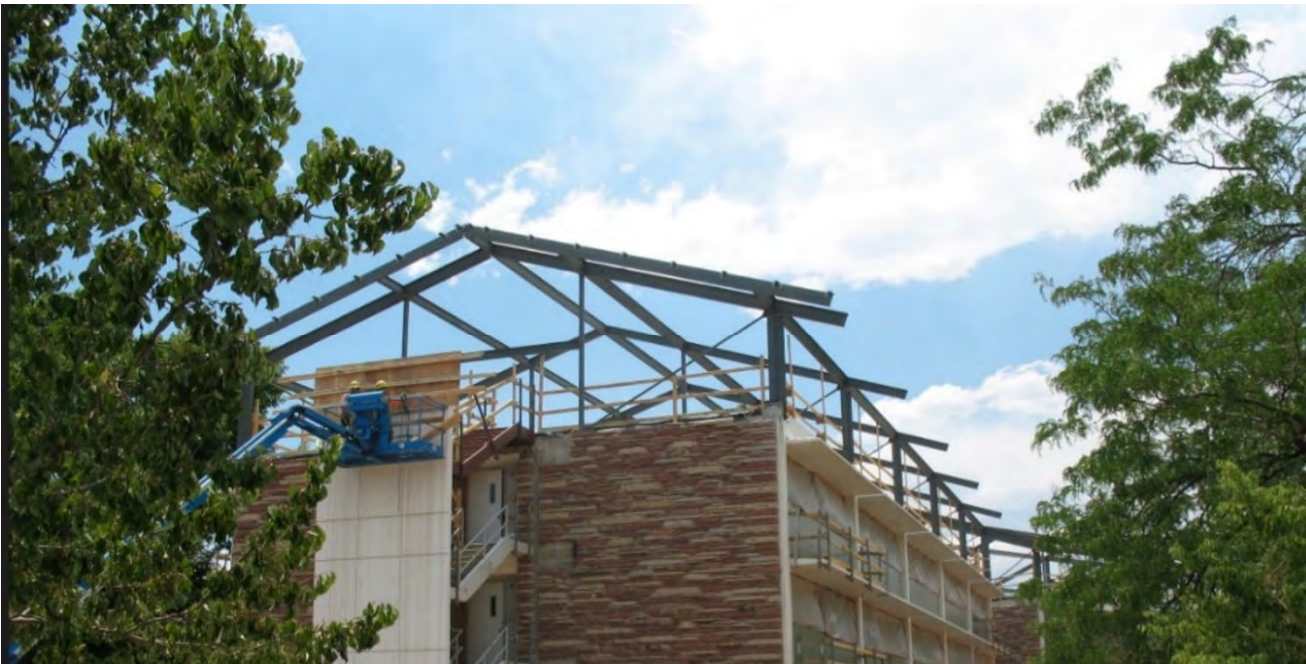
Parmelee Hall 4 th floor additions- steel roof structure construction – Braiden similar
