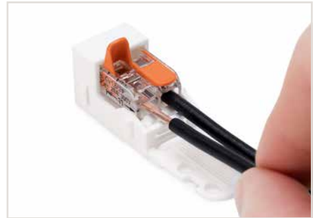
Inserting a conductor.
