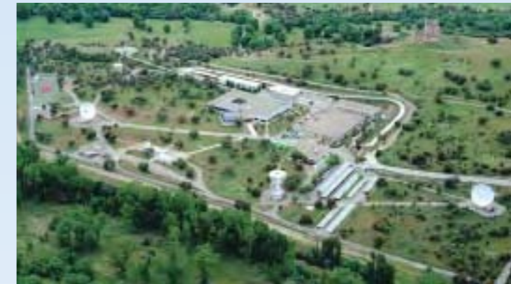
ESA's Villafranca tracking station near Madrid, Spain.
