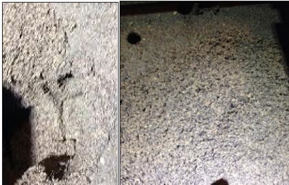
FIGURE 18. Pictures of mixed media found in Filter 4 bed during excavation.
